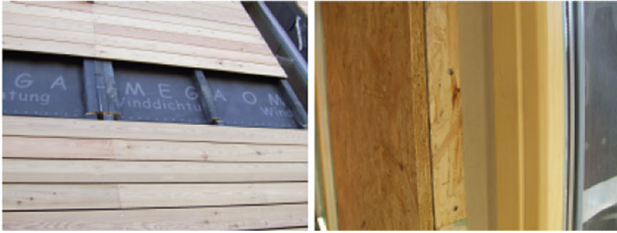
Fig. 2.14 Ventilated façade with a wooden cladding. A wind barrier is laid on top of the thermal insulation. The barrier must be water-vapour permeable to enable the transfer of water vapour without interstitial condensation (left). To ensure adequate air tightness of the building, all the joints between the doors or windows and the walls must be weatherstripped (right)
