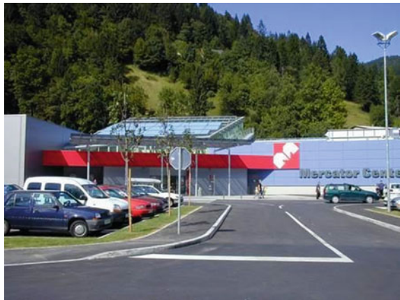
Fig. 4.76 The shopping mall with a useful floor area of 1500 m 2 is illuminated with skylights. The design illuminance level is 900 lx [36, 39]
