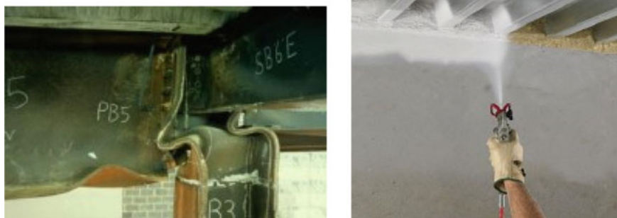
Fig. 6.7 Typical fire damage to an unprotected steel structure [7] (left); FireDam 200 coating is sprayed to improve the fire resistance of a steel building structure [8] (right)
