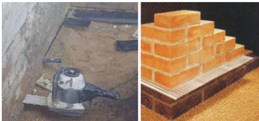
Fig. 3.12 Cutting the wall and inserting a bitumen strip (left) [12], inserted corrugated steel sheets (right) [12]
