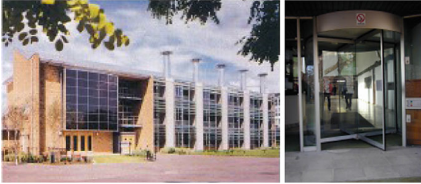
Fig. 2.9 Natural ventilation and building cooling by ventilation during the summertime can be enhanced with ventilation shafts (left) [Building Research Establishment, UK]. In contrast, to avoid large heat losses and discomfort, double slide or revolving doors are installed in tall buildings and staircases. In this way the inlet air-flow rate is reduced by up to 60% (for double slide doors) and by 98% in the case of revolving doors (right)
