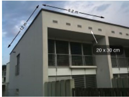
Fig. 1.48 Ventilation openings above the apartment ceiling. The same number of equally sized ventilation openings is also situated on the opposing north façade
