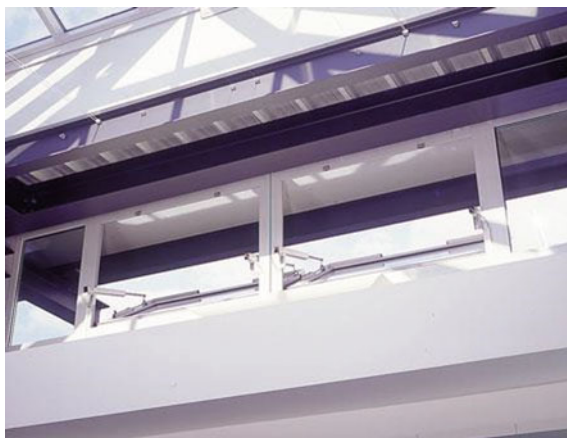
Fig. 6.29 Smoke flaps with automated opening mechanisms [24]
