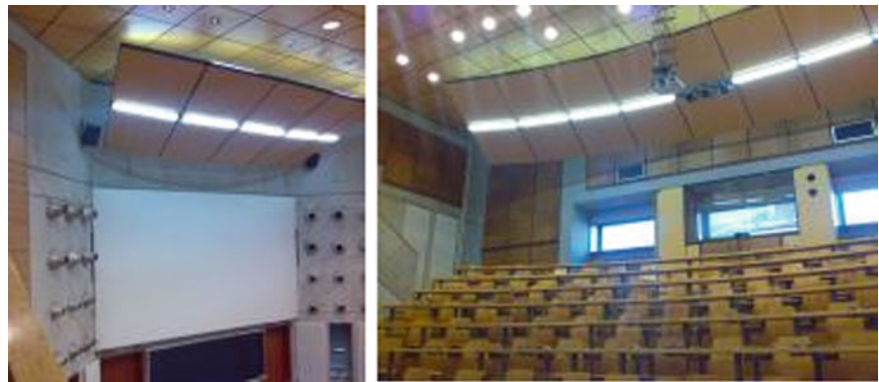
Fig. 5.45 With sound reflectors, we direct the sound wave emitted by the source to the listeners. Sound reflectors are usually flat or convex, so as not to create a condensed field of sound pressure in the room. Reflectors are placed above the sound source (left) and above more distant listeners (right)
